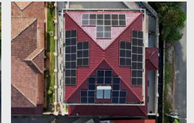
Bagan Serai, Perak 16.94kWp
