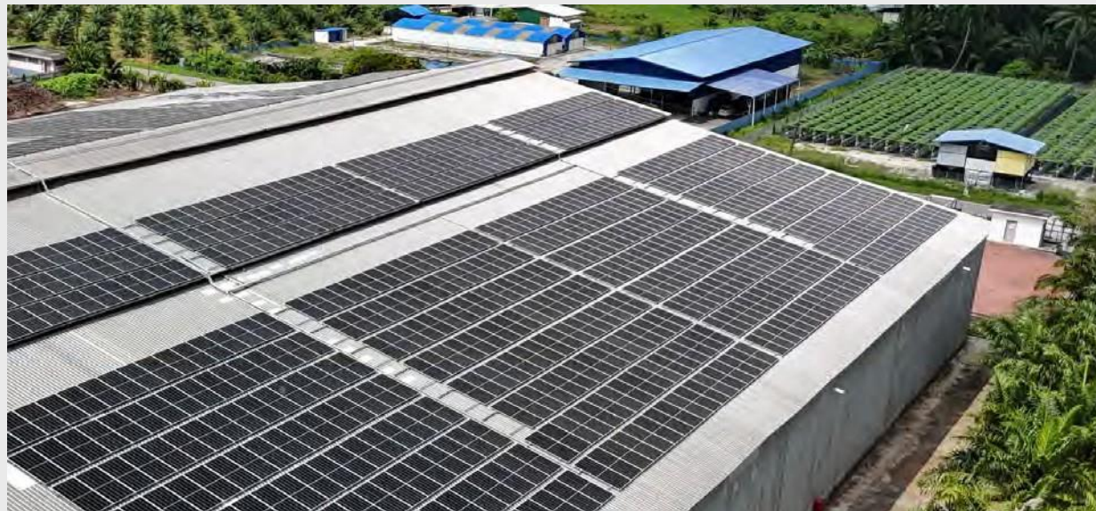
SUPREME KD PROCESSING SDN BHD [ Kiln-Drying & Steam Boiler Services ] 1.498MWp, Telok Panglima Garang, Selangor
